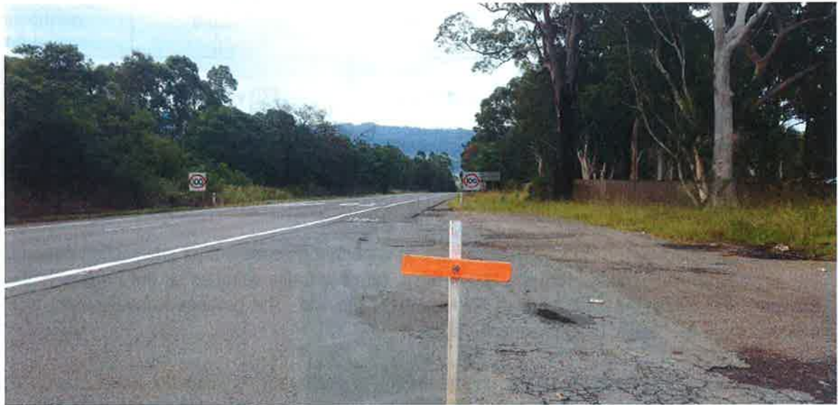
Sight distance looking north – 360m
